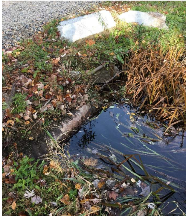
Existing Culvert Inlet
