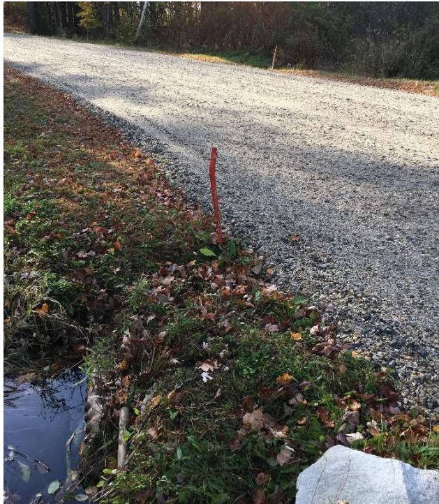
Existing Roadway Crossing
