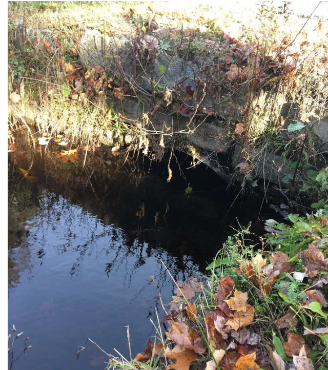
Existing Culvert Outlet
